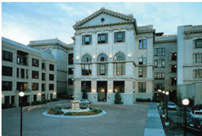
Mixed Use Redevelopment of Queen Anne High School in Seattle
